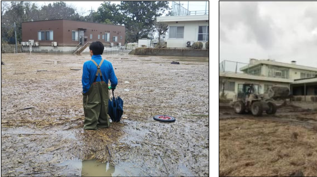
Fig 15 Left: The first author the day after the typhoon. The white building on the right is the residential facility and the brown building on the left is the consulting support office. Right: Bulldozer removing the straw.
