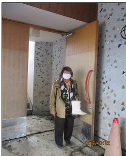
Fig.4 Yoshiko Abe, at the entrance of prefectural support center which is built with a raised floor. The headquarter of the corporation is settled on the third floor of this building for 6 months after flooding. The line above her head shows the height the water reached.
