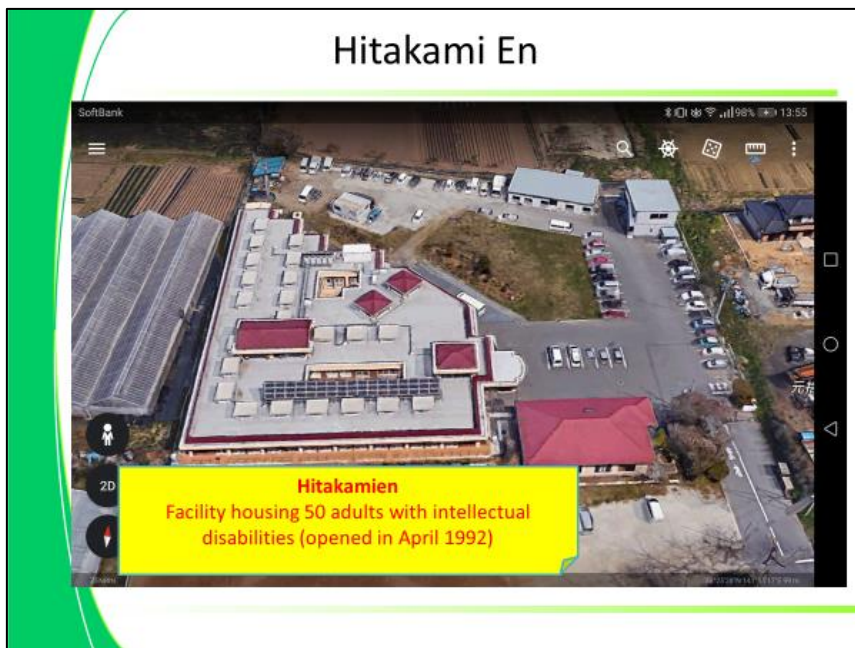
Figure 16 Full picture of Hitakamien which became a welfare evacuation center
