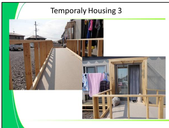
Figure 27 Ramp installed at the entrance to a room at the back of temporary housing
