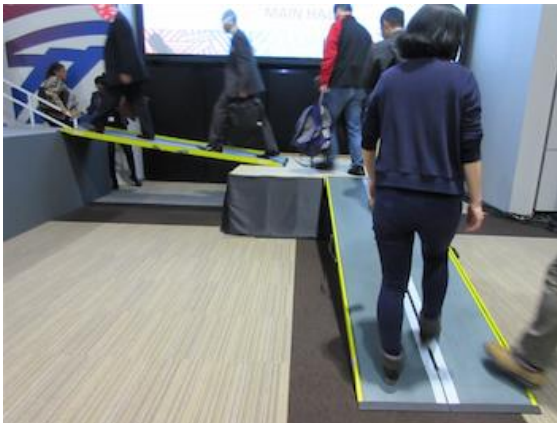
Fig.3 Two long ramps were combined to make access to the high main stage for wheelchair users.
